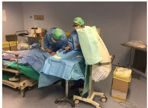
Operio focused laminar flow is the ideal solution for ophthalmology and intravitreal injections. The flow does not pass obstacles such as the surgical microscope and the head-neck area of the operating surgeon maintaining an extreme high degree of asepsis. Intravitreal injections can also be prepared outside the normal operating room in combination with operio. Operio creates a higher degree of asepsis than any conventional operating room for two reasons:
